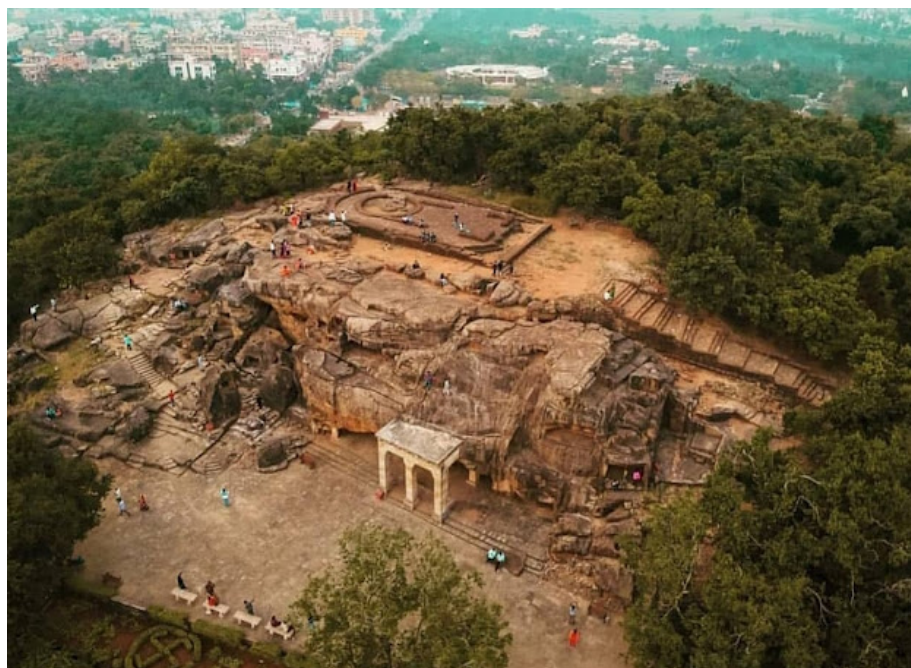
Top view of the Apsidal Chaitya structure at Udaygiri
